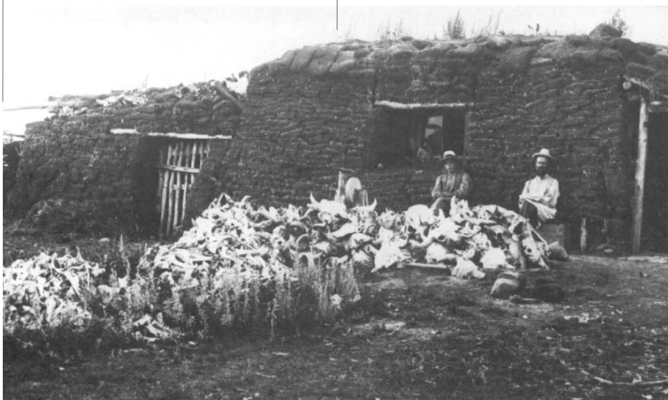
This is a much less romantic view of the conditions faced by the prairie settlers. The hut is constructed entirely of blocks of tough sod, chopped from the surrounding landscape. The bleached buffalo bones, collected for hundreds of miles across the plains, could be sold through the CPR to Minneapolis where they fetched seven dollars a ton.
